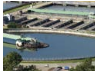
Municipal or industrial wastewater tertiary treatment
